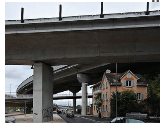
A house beneath a bridge in Zurich, Switzerland. The bridge was constructed over the house after the owner refused to leave.
